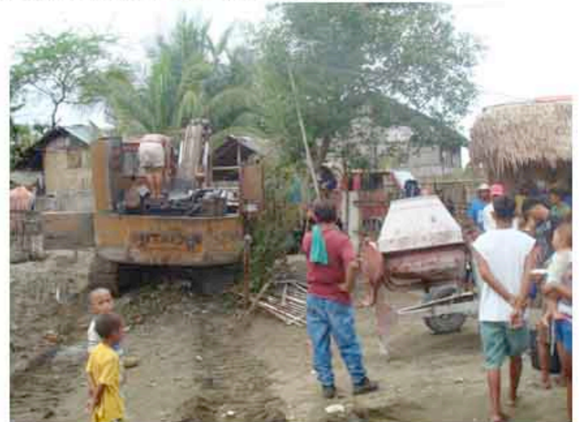
The forkcrane getting ready to demolish the fence and the church
